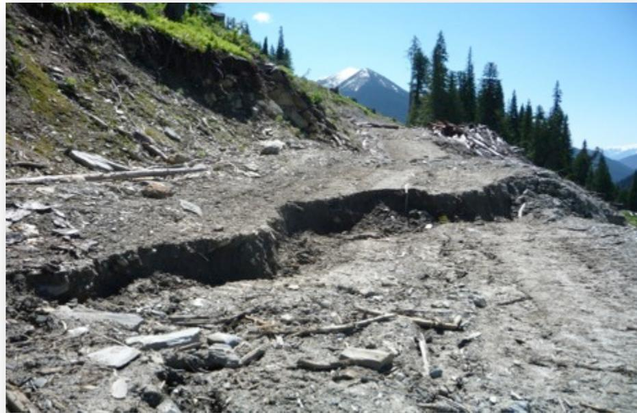
Road Maintenance – failure of a road prism. Road under permit but considered a wilderness road. Still utilized by public. No warning signs and failure of the culvert below introduced sediment into an S4 fish stream.
