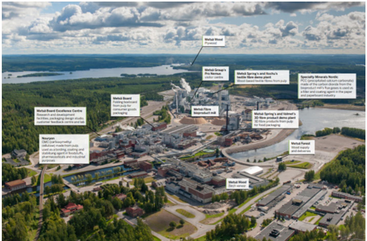
Metsa's integrated bioprocessing site includes a large modern pulpmill, birch peeler plant, sawmill, board plant, bioenergy plant, and several bioproduct facilities.
