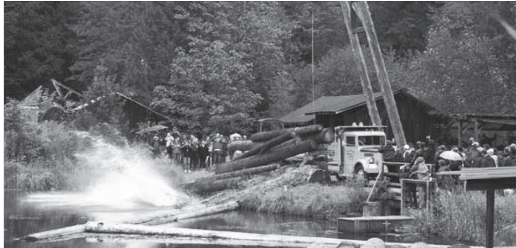
Historic McLean "Steam" Mill, 2007 AGM Port Alberni
